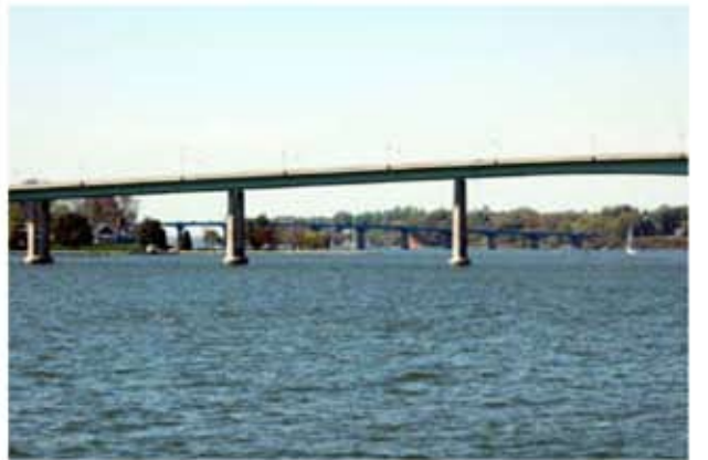
Severn River Bridge, Annapolis, Maryland
