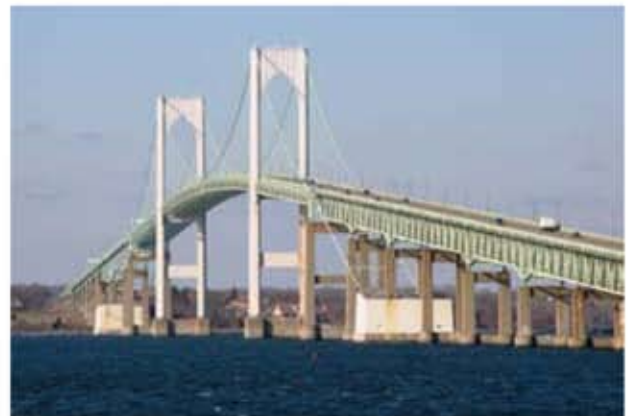
Newport, Rhode Island Bridge
