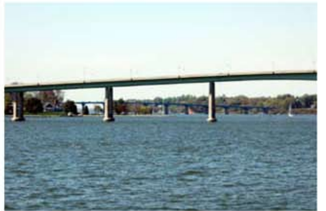
Severn River Bridge, Annapolis, Maryland
