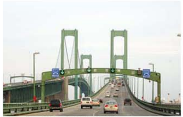
Delaware Memorial Bridge, Wilmington, Delaware
